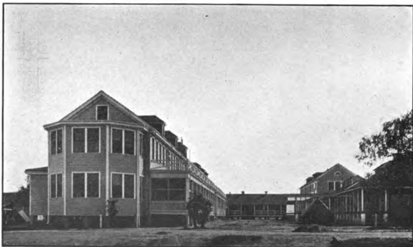
Emergency hospital buildings, Marine Barracks, Parris Island, S. C., showing wards and solarium.
