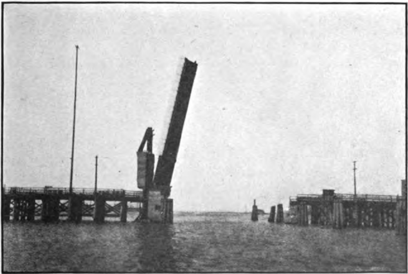
Causeway connecting Mare Island Navy Yard with mainland; bascule bridge raised.
