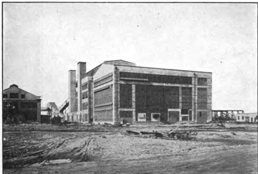
Generator-room end of power plant, Navy Yard, Philadelphia, Pa.
