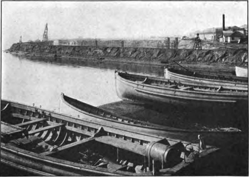
Filling operation in progress, Navy Yard, Puget Sound, Wash.
