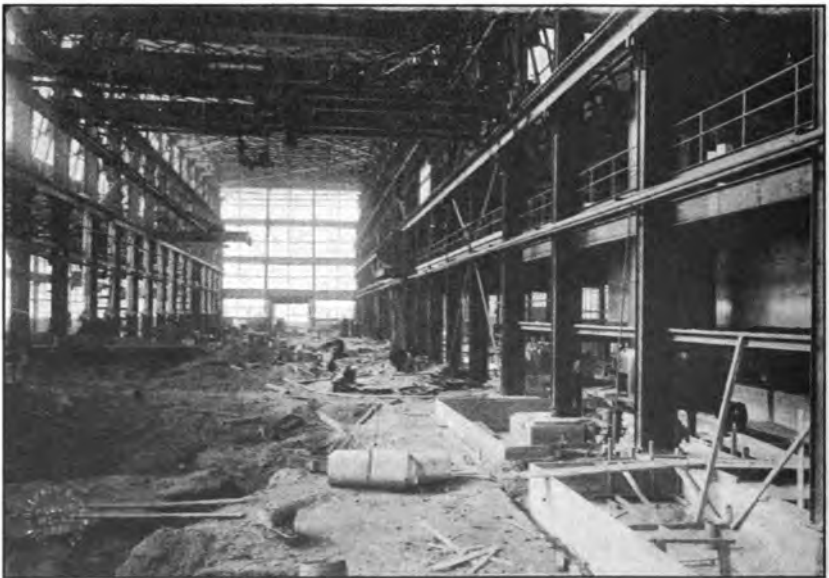
Foundry, Navy Yard, Philadelphia, Pa. Interior view.
