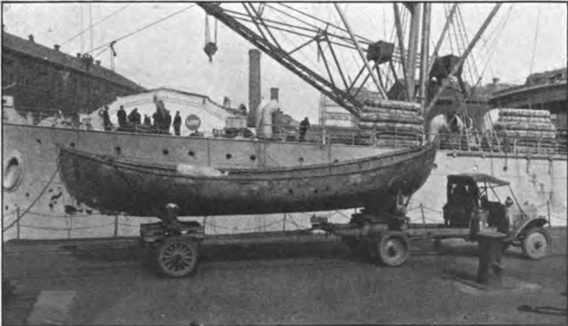
Adaptation of yard truck and semi-trailer for boat haulage. 37022—21—31
