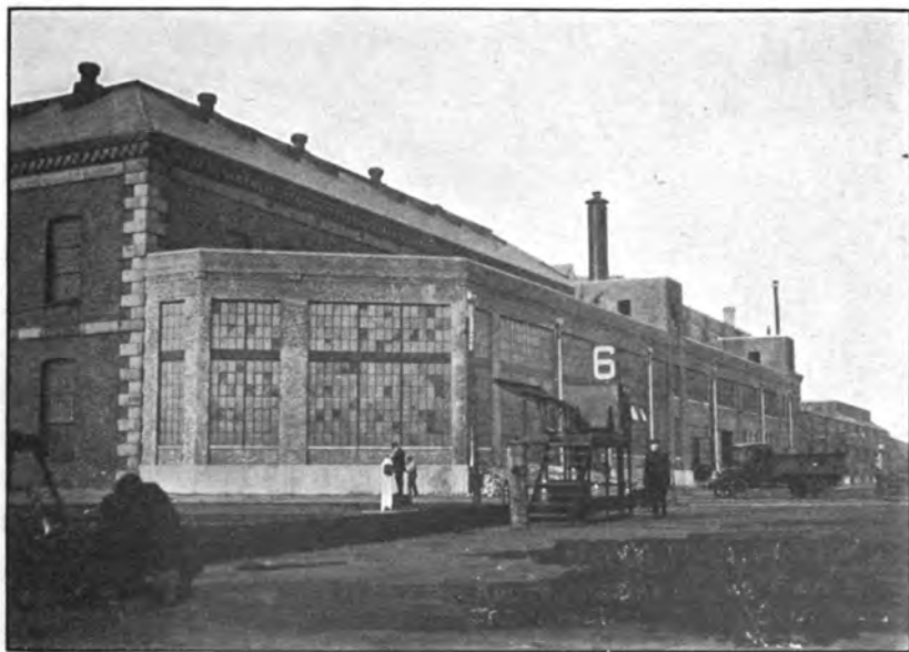
Foundry, Navy Yard, Boston, Mass. Second extension.
