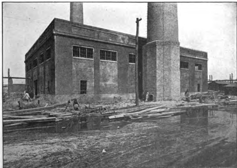
Boiler plant, East Camp, Hampton Roads, Va.
