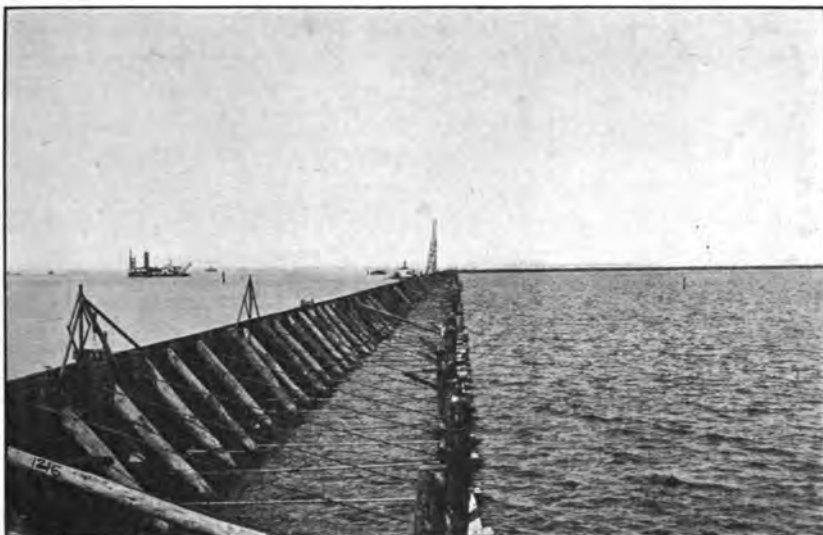
West bulkhead before filling, Naval Operating Base, Hampton Roads, Va.
