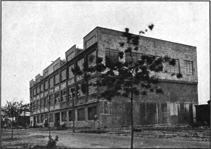
Pattern shop and storage building, Navy Yard, Philadelphia, Pa.
