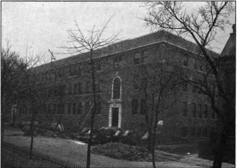
Steam Engineering School, Stevens Institute, Hoboken, N. J.
