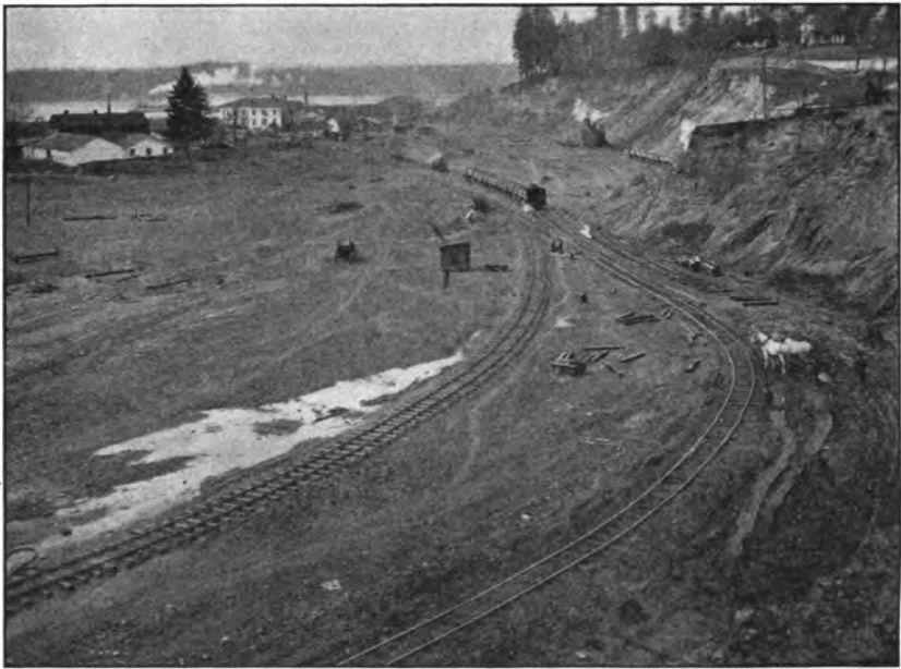
Grading and filling operations, Navy Yard, Puget Sound, Wash. General view.
