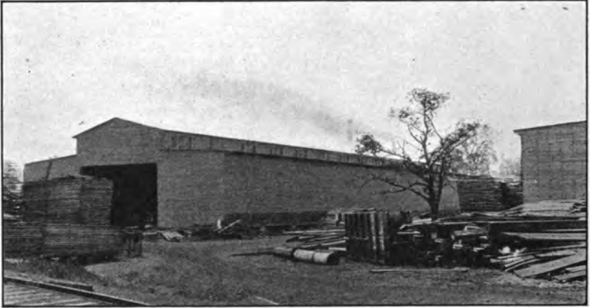
Lumber-storage building, Navy Yard, Portsmouth, N. H.
