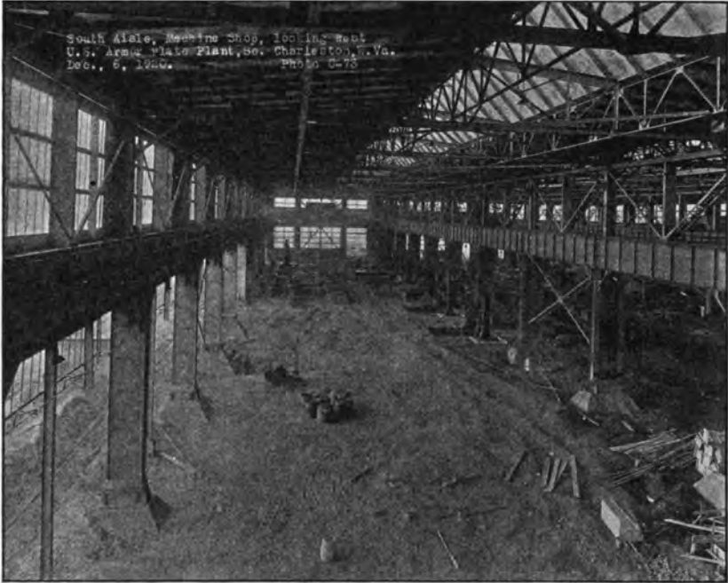
South aisle of machine shop, Armor Plant, Charleston, W. Va.
