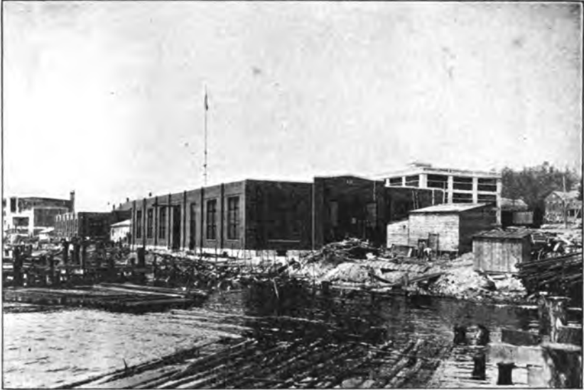
Battery-overhaul building, Submarine Base, New London, Conn.
