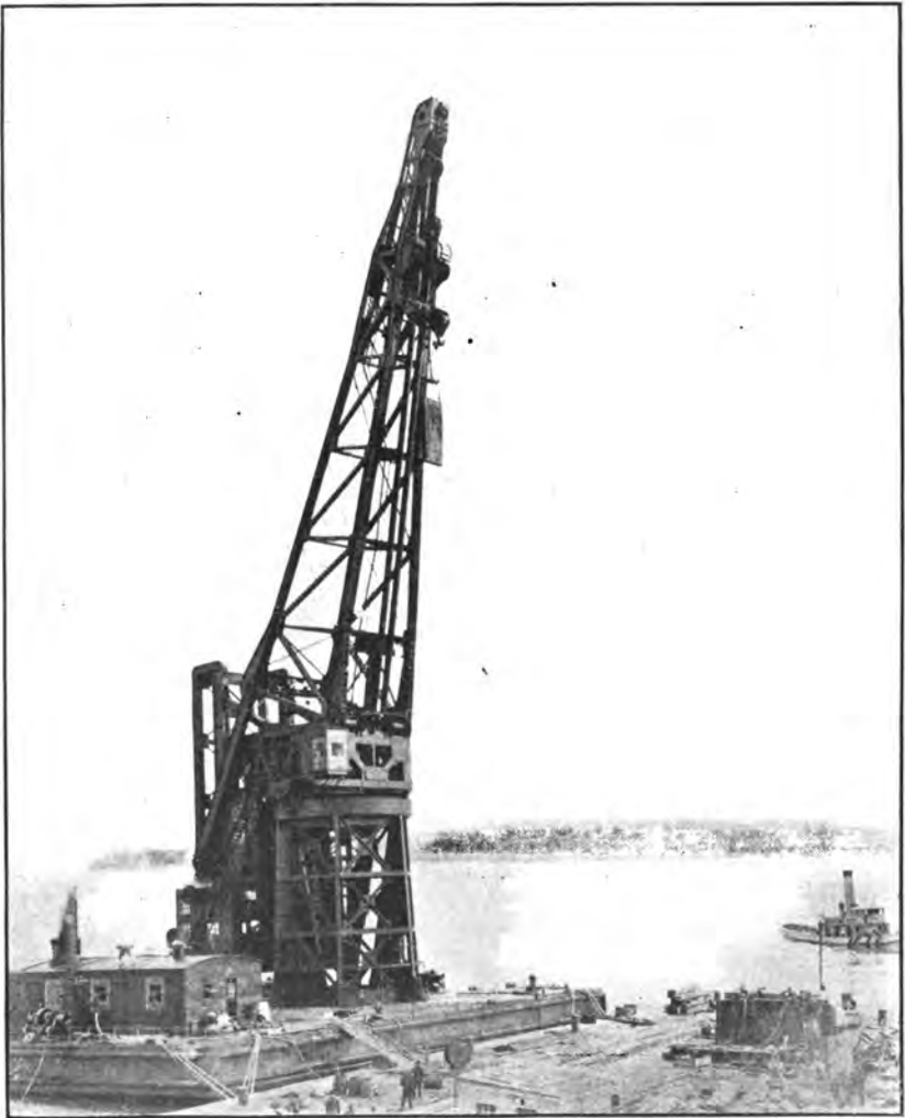
Floating crane (150-ton), Navy Yard, Mare Island, Calif.
