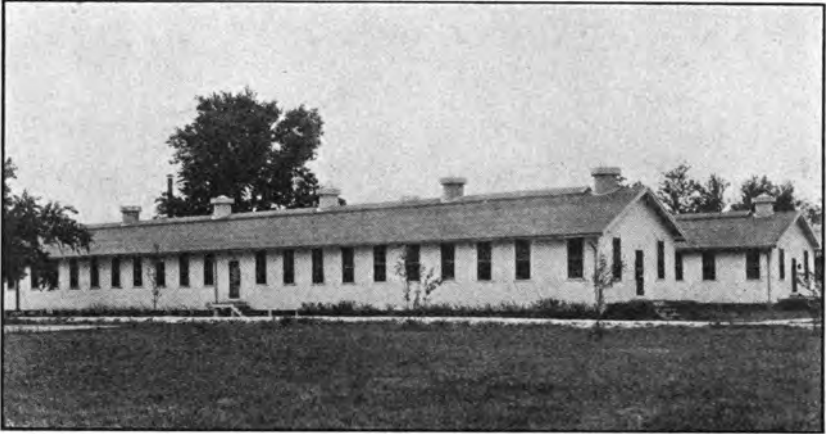
Ward buildings, Naval Hospital, New Orleans, La.
