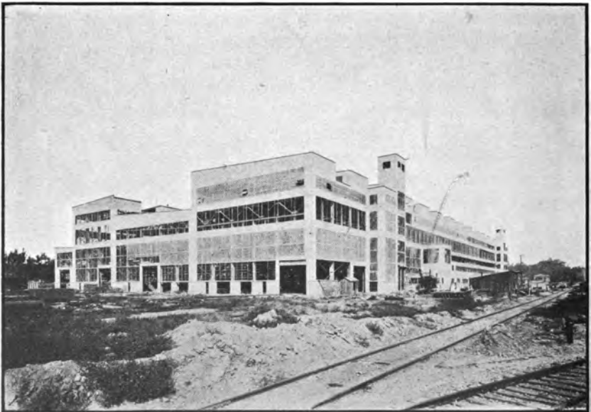
Structural shop, Navy Yard, Mare Island, Calif.
