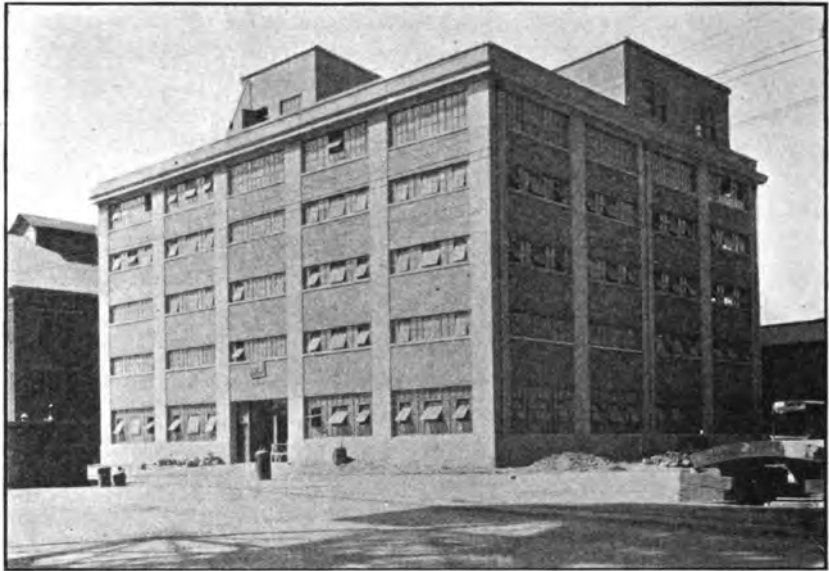
Electrical storehouse, Navy Yard, Mare Island, Calif.
