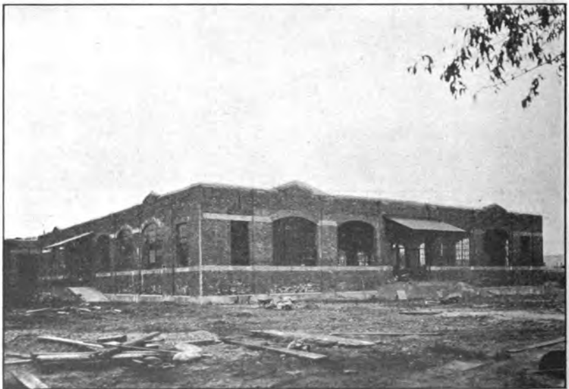
Advance-base storehouse for Marine Corps, Navy Yard, Philadelphia, Pa.
