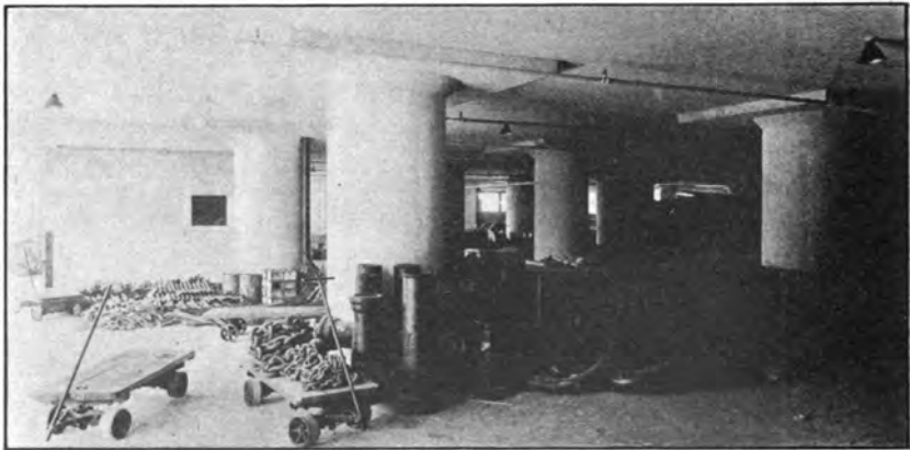
General storehouse, Navy Yard, Puget Sound, Wash. Interior view, ground floor.
