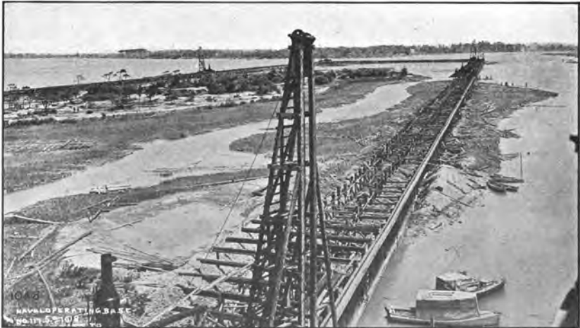
Bulkheads for aviation pier, Naval Operating Base, Hampton Roads, Va.
