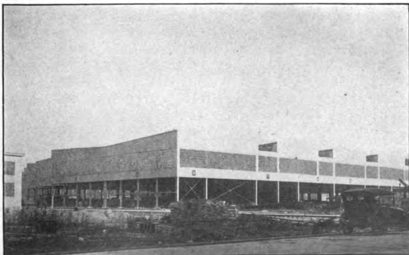
Steel-storage shed, Navy Yard, Norfolk, Va.
