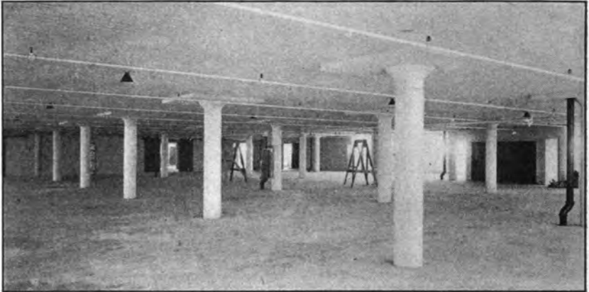
General storehouse, Navy Yard, Puget Sound, Wash. Interior view, top floor.
