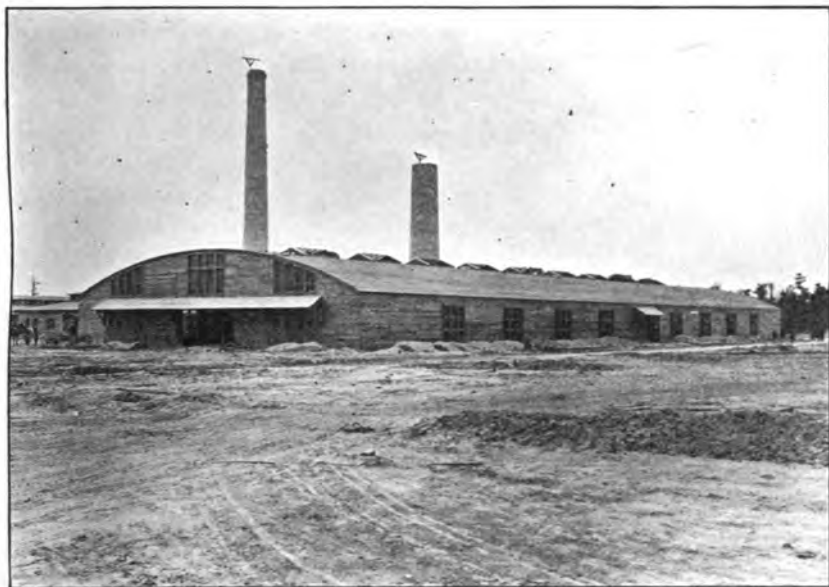
Drill hall at East Camp, Hampton Roads, Va.
